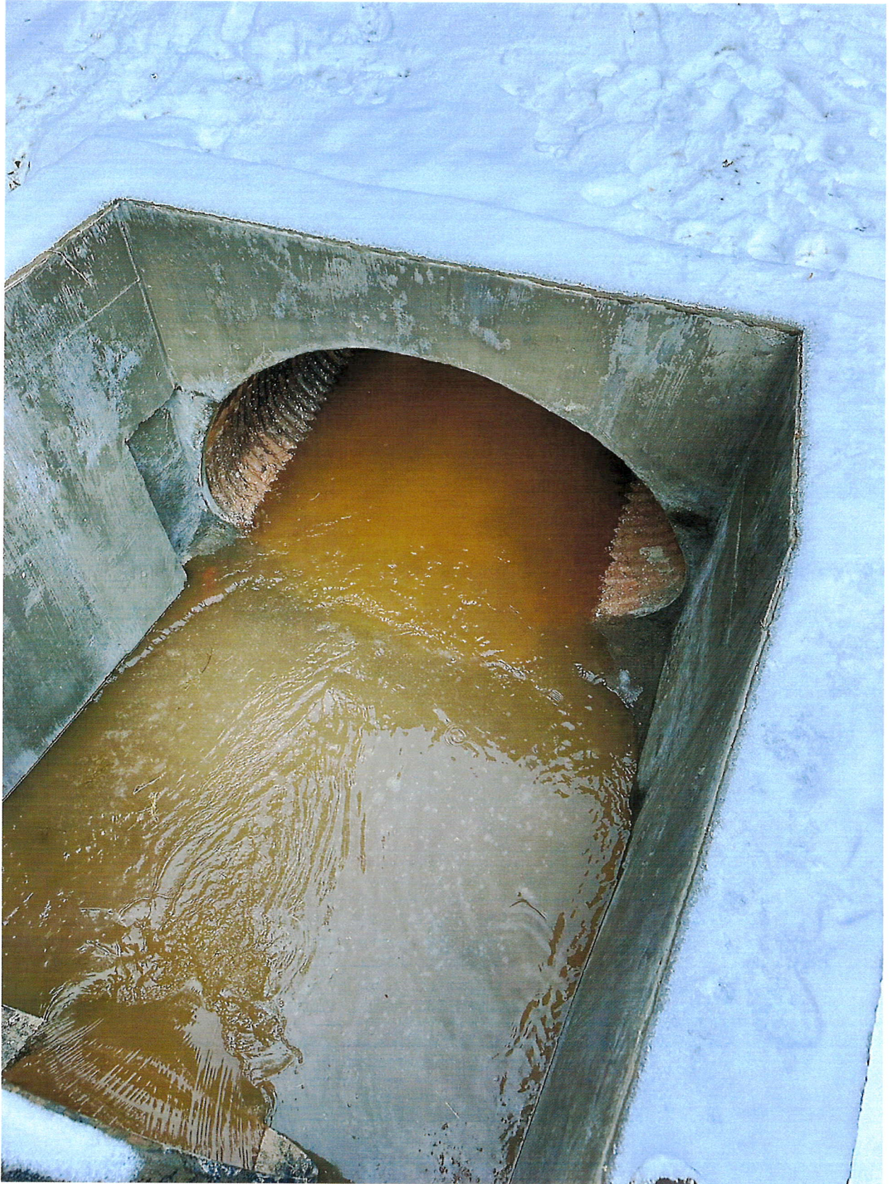
Hell 4 Stout Flume, is now the Hell 4 Stout Siphon
