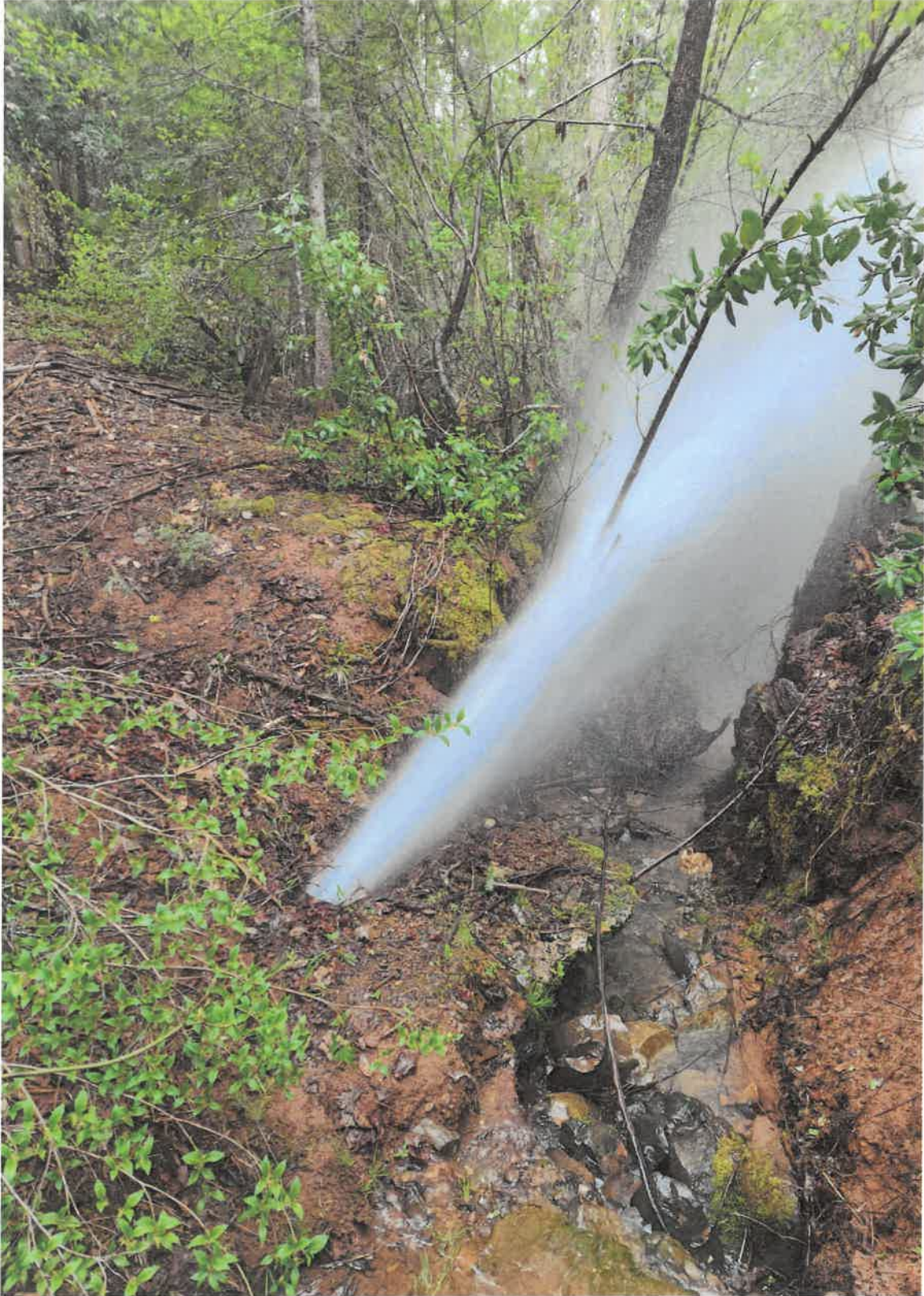
Mail Line Break- After being necked down for repair
