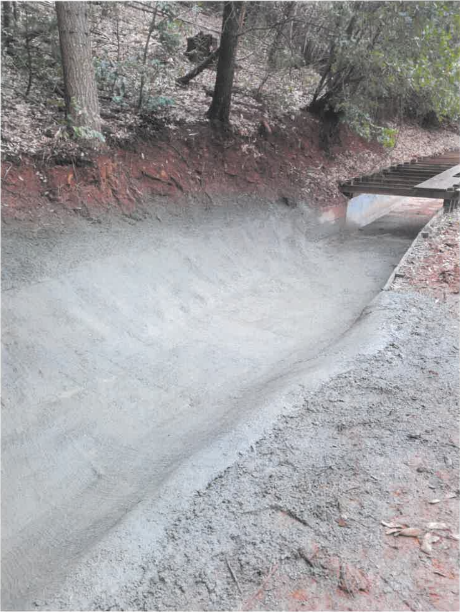
Upper Forbestown Ditch
